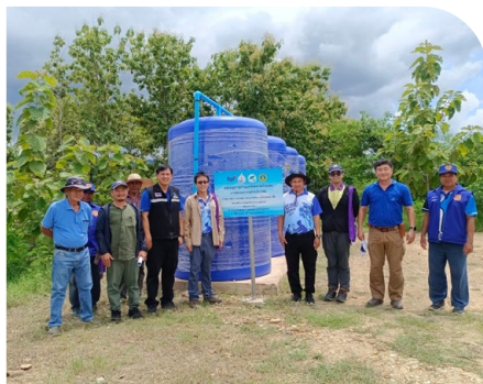
▲ Water reservoir tank, Tambon Nam Lao, Amphoe Rong Kwang, Phrae Province
